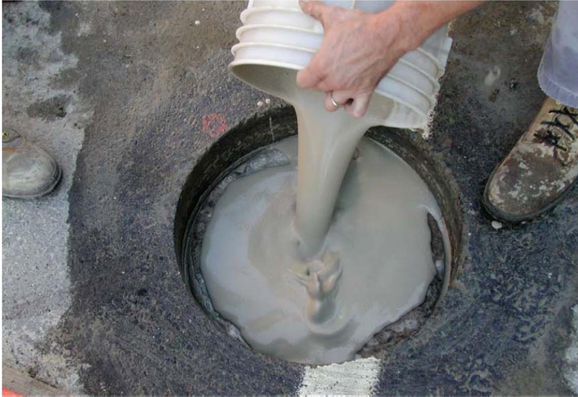
Figure 5.15. Grout poured into keyhole on top of PCC delaminated segment
