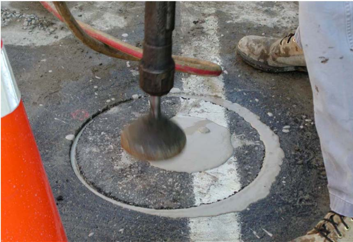
Figure 5.16. AC core tamped into place
