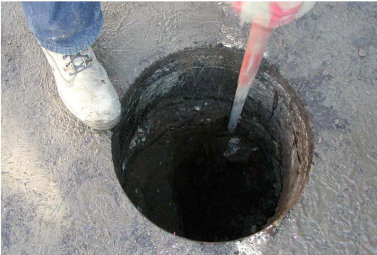
Figure 5.12. Manual steering of material in the keyhole to promote pumping action
