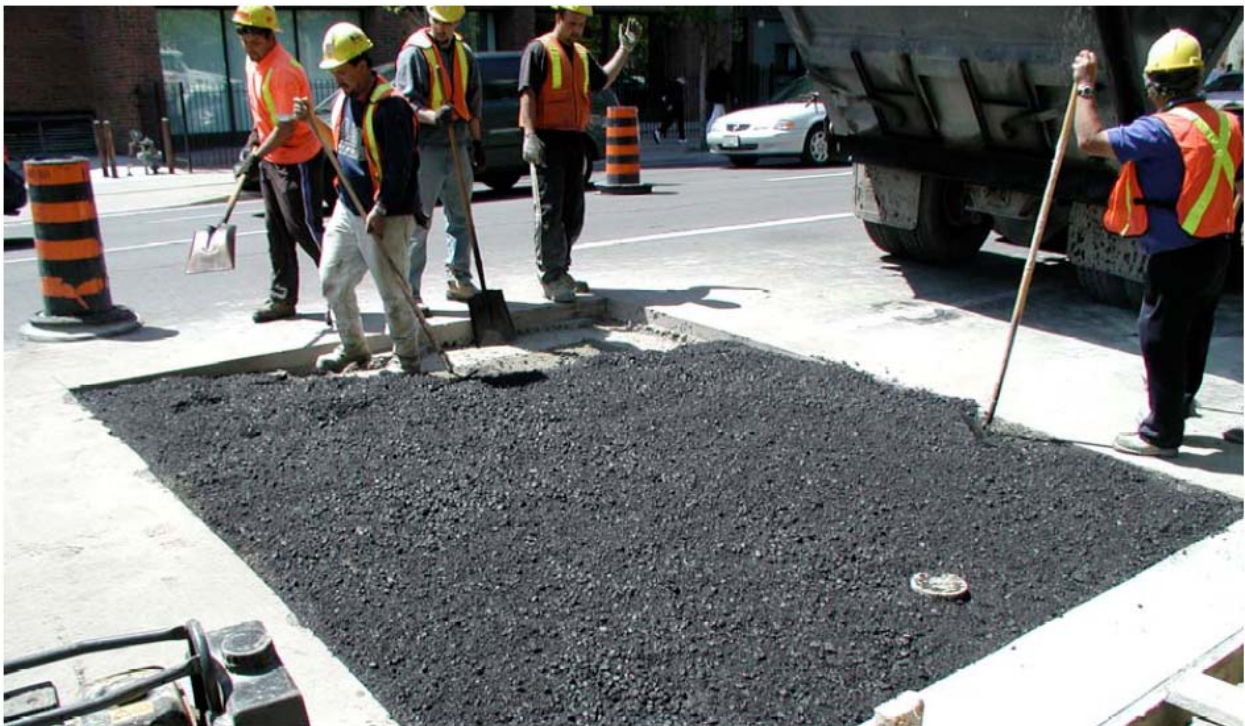
Figure 5.8. Placement of the HL8 layer on top of the PCC base
