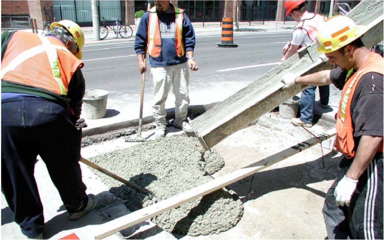
Figure 5.7. Casting of PCC base
