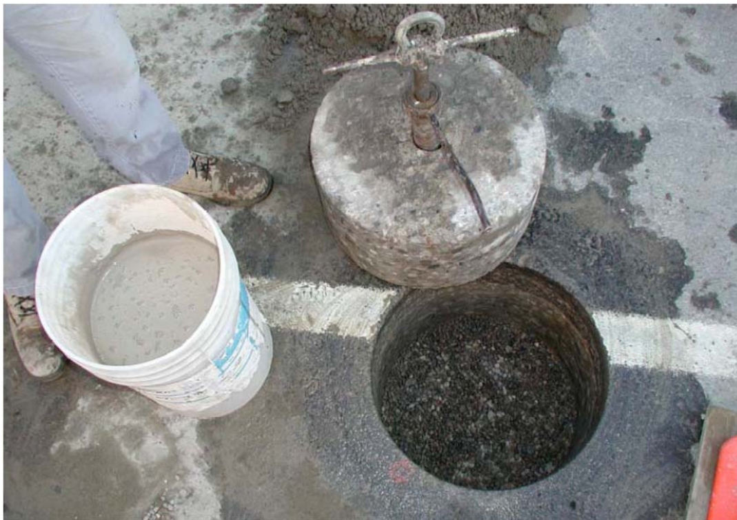
Figure 5.14. Water drained from unshrinkable fill and grout ready for application
