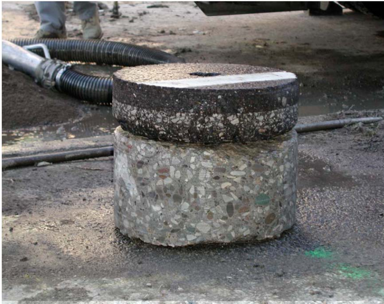
Figure 5.10. Original core recovered by coring and used later to restore the keyhole
