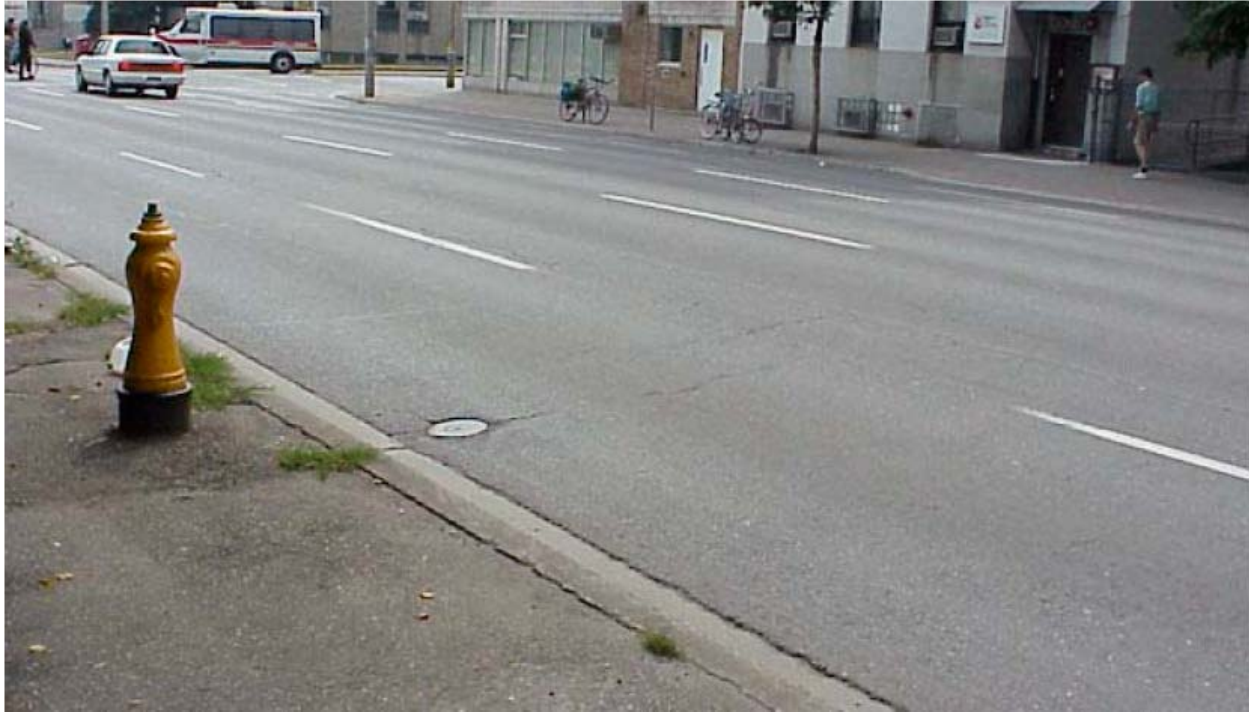
Figure 2.2. Site on Jarvis Street
