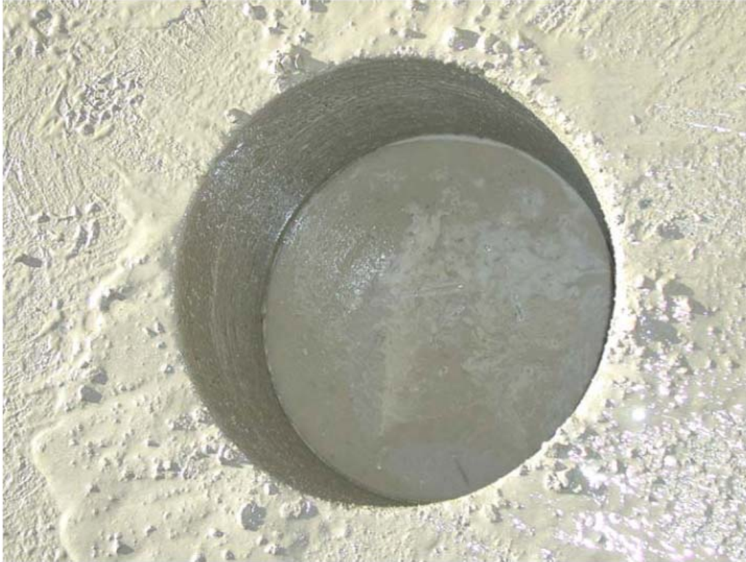
Figure 5.13. Freshly poured unshrinkable fill
